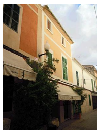
C/ Major, 84 - Nivell: b.3
