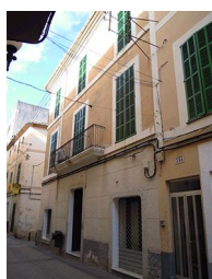
C/ Major, 37 - Nivell: b.3
