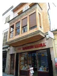
C/ Major, 25 - Nivell: b.3
