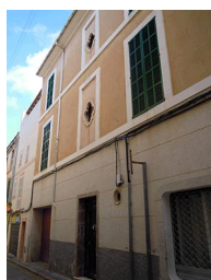
C/ Major, 37 - Nivell: b.3
