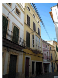
C/ Major, 46 - Nivell: b.2
