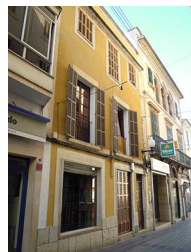
C/ Major, 30 - Nivell: b.2.3
