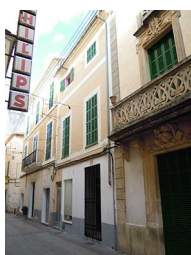
C/ Major, 39 - Nivell: b.3
