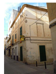
C/ Major, 35 - Nivell: b.3
