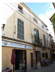
C/ Major, 21 - Nivell: b.3
