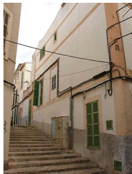
C/ Major, 13 - Nivell: b.2.3
