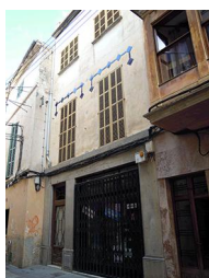
C/ Major, 23 - Nivell: b.2.3
