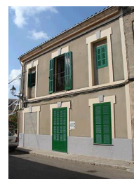
C/ Major, 22 - Nivell: b.2.3
