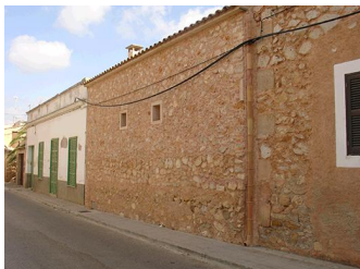
C/ Major, 31 (1) - Nivell: b.1.2
