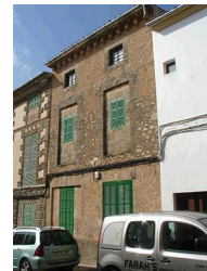
C/ Major, 6 - Nivell: b.2.3
