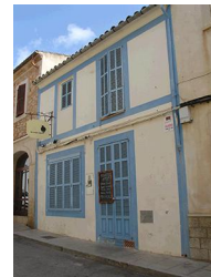
C/ Major, 7 - Nivell: b.2.3
