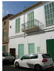
C/ Major, 4 - Nivell: b.2.3
