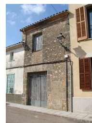
C/ Major, 28 (2) - Nivell: b.2
