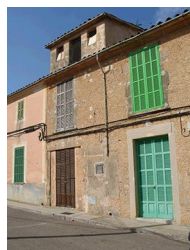
C/ Major, 38 - Nivell: b.1.2
