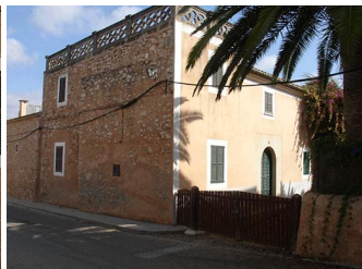
C/ Major, 31 (2) - Nivell: b.2
