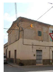
C/ Major, 11 - Nivell: b.2.3
