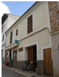
C/ Major, 3 - Nivell: b.2
