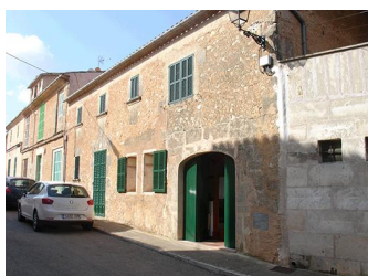
C/ Major, 34 - Nivell: b.2
