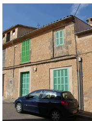
C/ Major, 36 - Nivell: b.2
