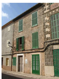
C/ Major, 10 - Nivell: b.3
