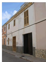
C/ Major, 19 - Nivell: b.3
