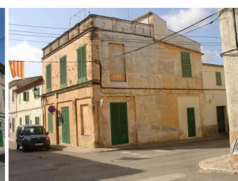
C/ Major, 14 - Nivell: b.2
