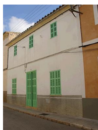
C/ Major, 15 - Nivell: b.2.3
