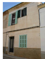
C/ Major, 13 - Nivell: b.2.3
