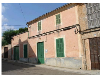
C/ Major, 40 - Nivell: b.2
