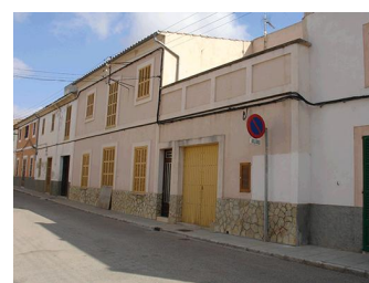
C/ Major, 21 - Nivell: b.1.3
