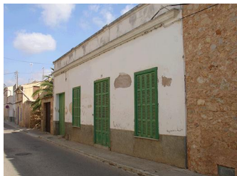
C/ Major, 29 - Nivell: b.1.3
