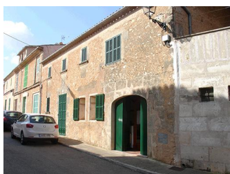
C/ Major, 34. Nivell: b.2
