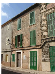
C/ Major, 10. Nivell: b.3
