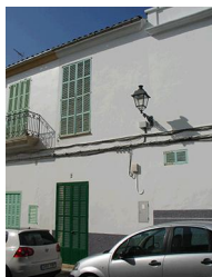
C/ Major, 2. Nivell: b.3
