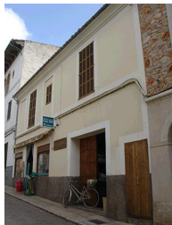
C/ Major, 3. Nivell: b.2
