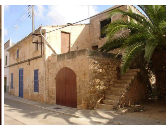
C/ Major, 25 (2). Nivell: b.1
