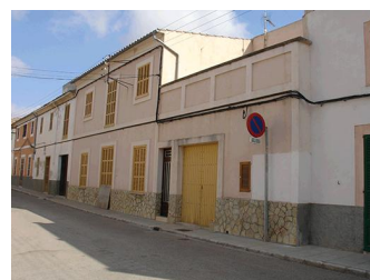
C/ Major, 21. Nivell: b.1.3
