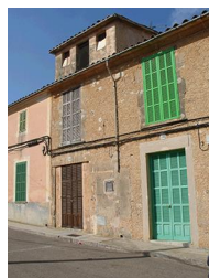
C/ Major, 38. Nivell: b.1.2
