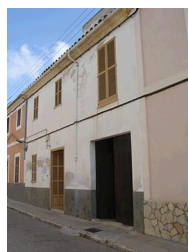
C/ Major, 19. Nivell: b.3
