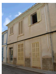
C/ Major, 9. Nivell: b.2.3
