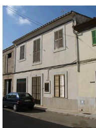
C/ Major, 18. Nivell: b.3
