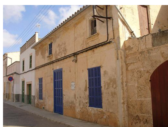
C/ Major, 25 (1). Nivell: b.2
