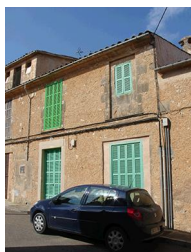
C/ Major, 36. Nivell: b.2
