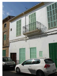
C/ Major, 4. Nivell: b.2.3
