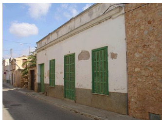
C/ Major, 29. Nivell: b.1.3
