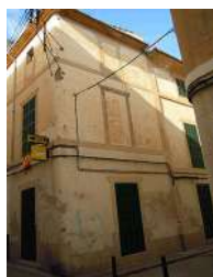
C/ Major, 35. Nivell: b.2
