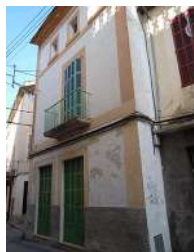
C/ Major, 13. Nivell: b.3
