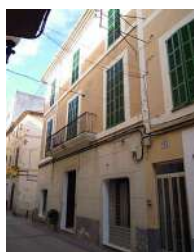
C/ Major, 37. Nivell: b.3
