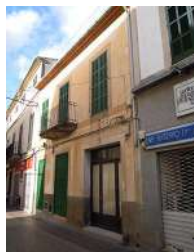
C/ Major, 47. Nivell: b.1
