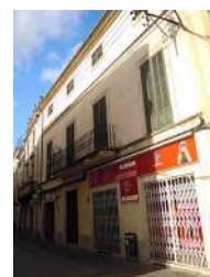
C/ Major, 43-45. Nivell: b.3
