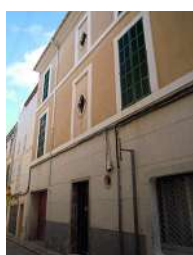
C/ Major, 37. Nivell: b.3
